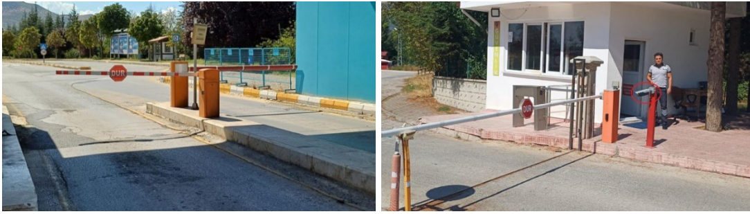
Automated vehicle identification and gate system at the entrances of Tokat Gaziosmanpaşa University
