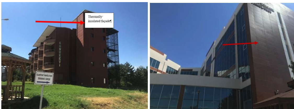
Thermally insulated façade, an example from the TOGU Guesthouse (left) and an example from a faculty building (right)
