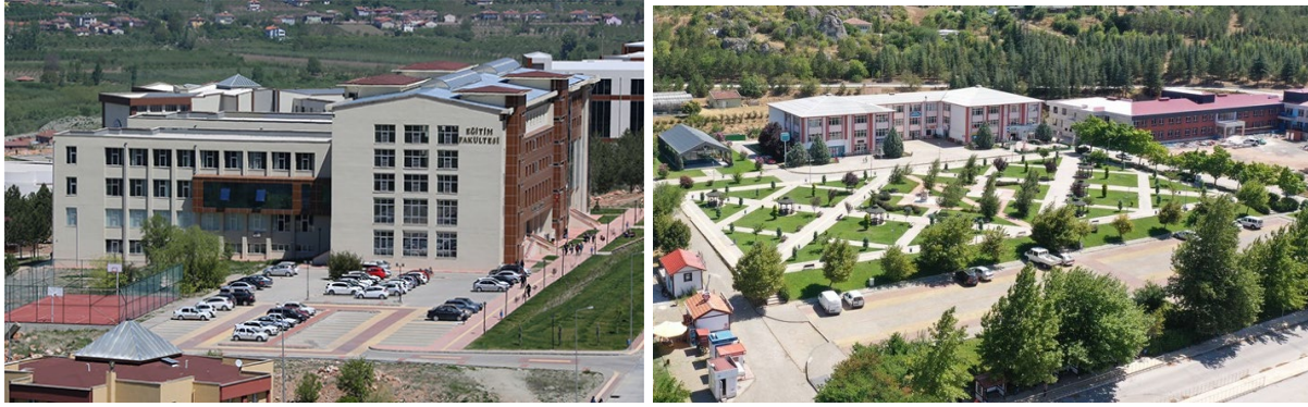
Examples of parking areas on main campus
