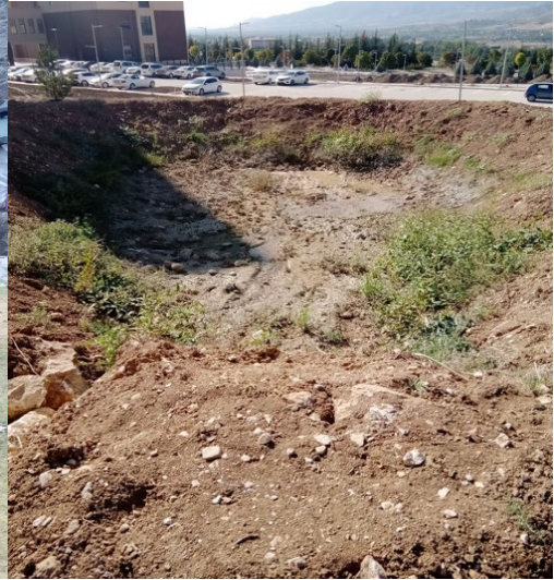
Rectorate Building water collection pond
