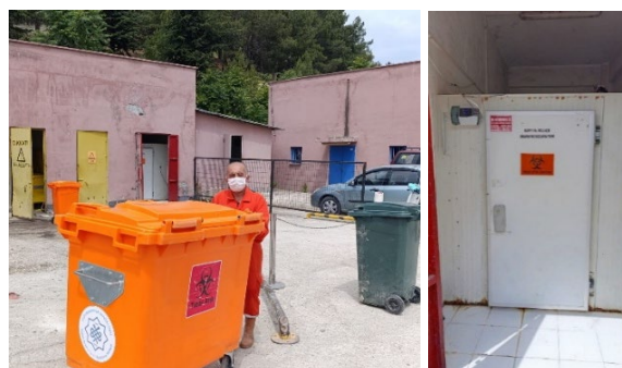
Toxic waste treatment system of TOGU university hospital
