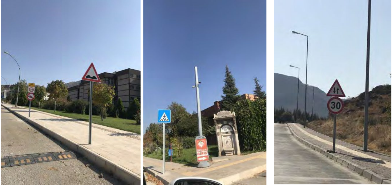
Traffic signs and monitoring system
