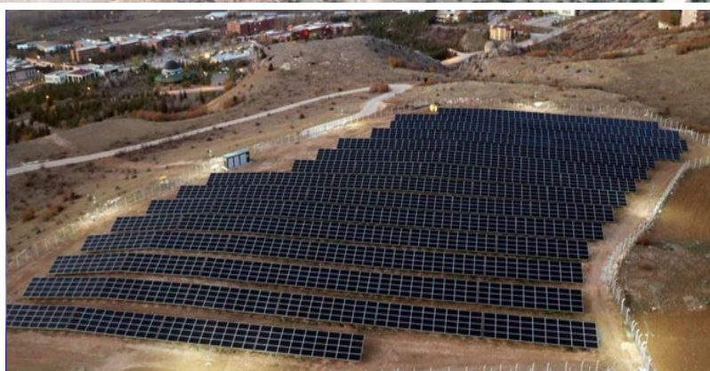
Existing and newly installed solar power plants (SPPs) on campus
